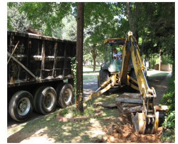
Defective concrete is removed
