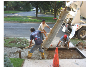
New concrete is poured into forms
