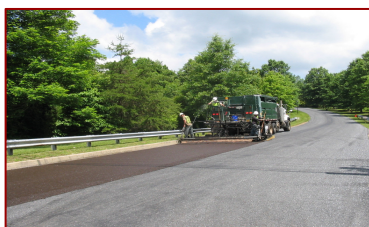
Micro surfacing application
