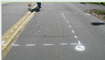
Typical survey paint markings
