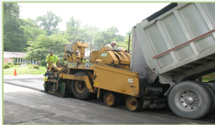
Typical hot mix asphalt paving operation
