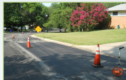
New patch is flush with existing pavement
