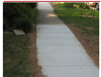
Completed sidewalk repair
