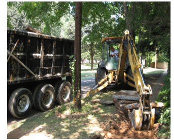
Defective concrete is removed
