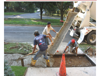
New concrete is poured into forms
