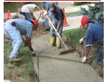
Concrete is smoothed and finished
