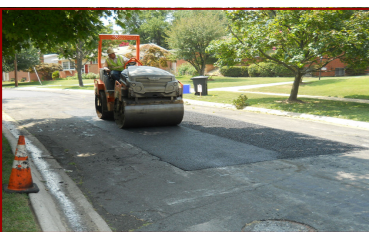
Distressed areas will be patched prior to resurfacing
