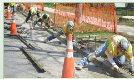
Concrete is smoothed and finished
