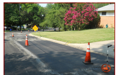
New patch is flush with existing pavement
