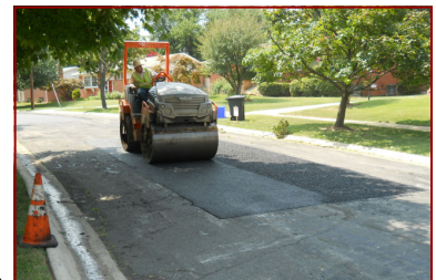
New asphalt is placed and compacted
