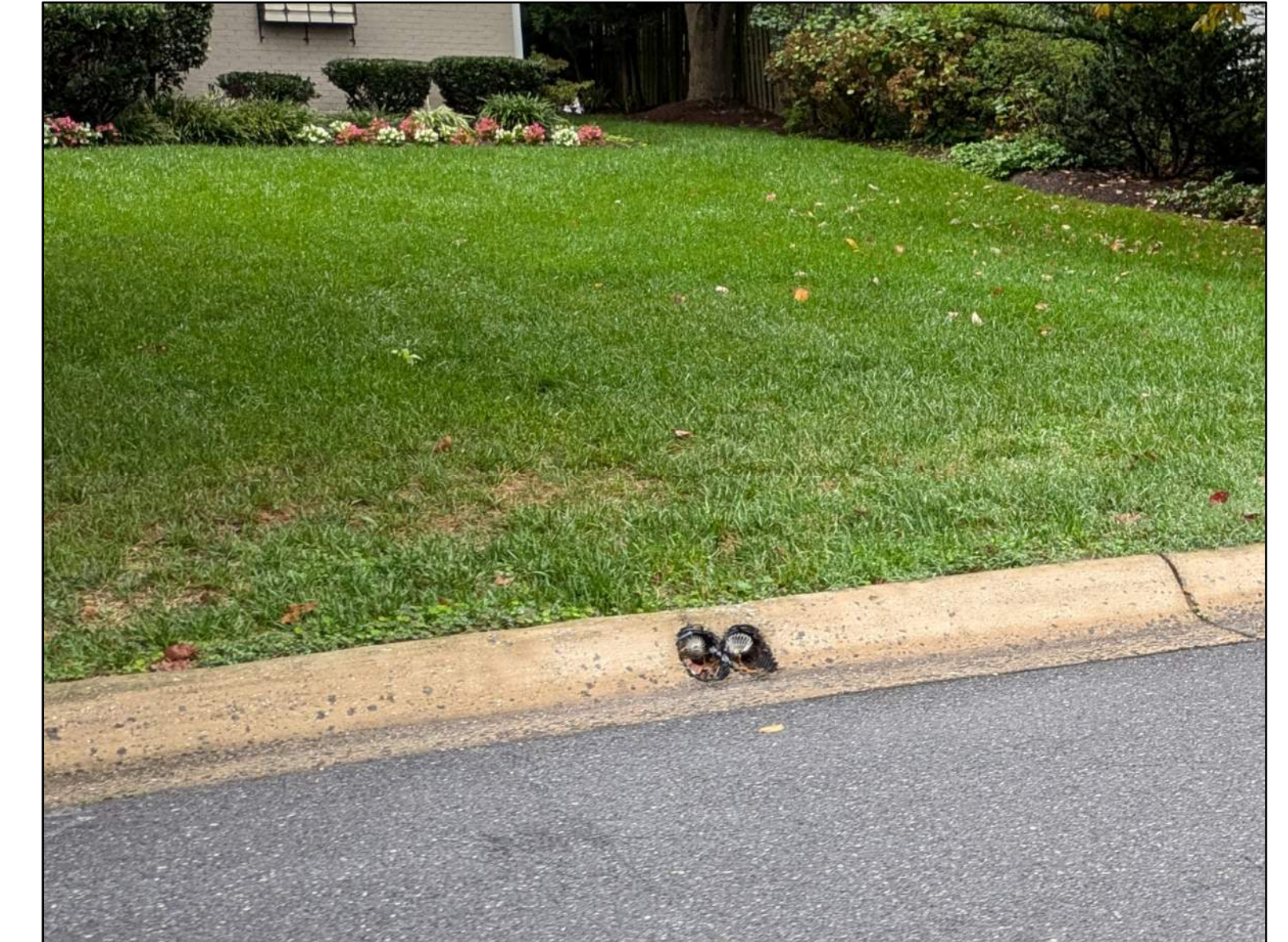
Properties with downspout outfalls through curb.
