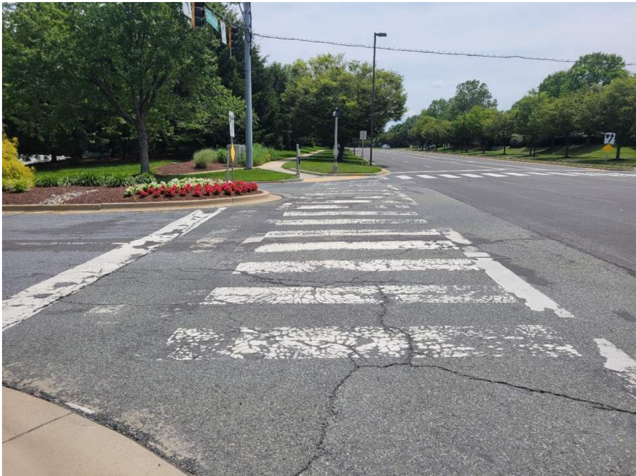
Photo 1. Taken from northwest corner looking eastbound along Observation Dr at the north leg crossing. Poor pavement marking condition.
