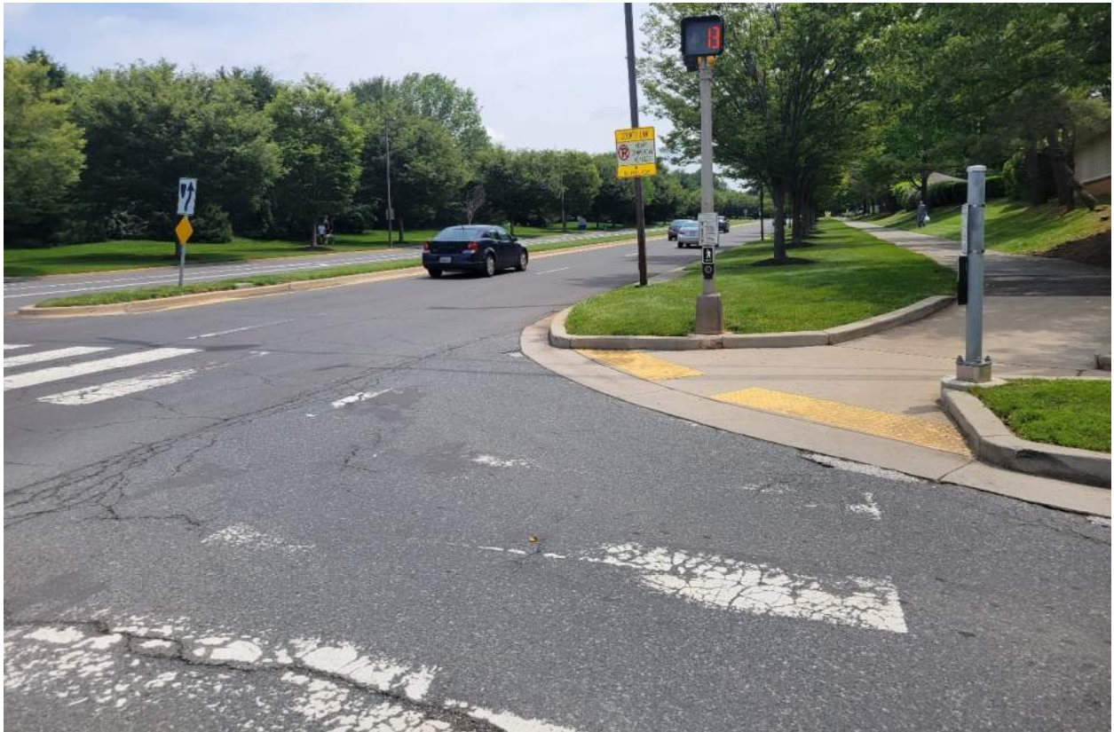
Photo 3: All pedestrian ramps consist of two detectable warning surfaces that do not guide motorists perpendicular to the roadway.
