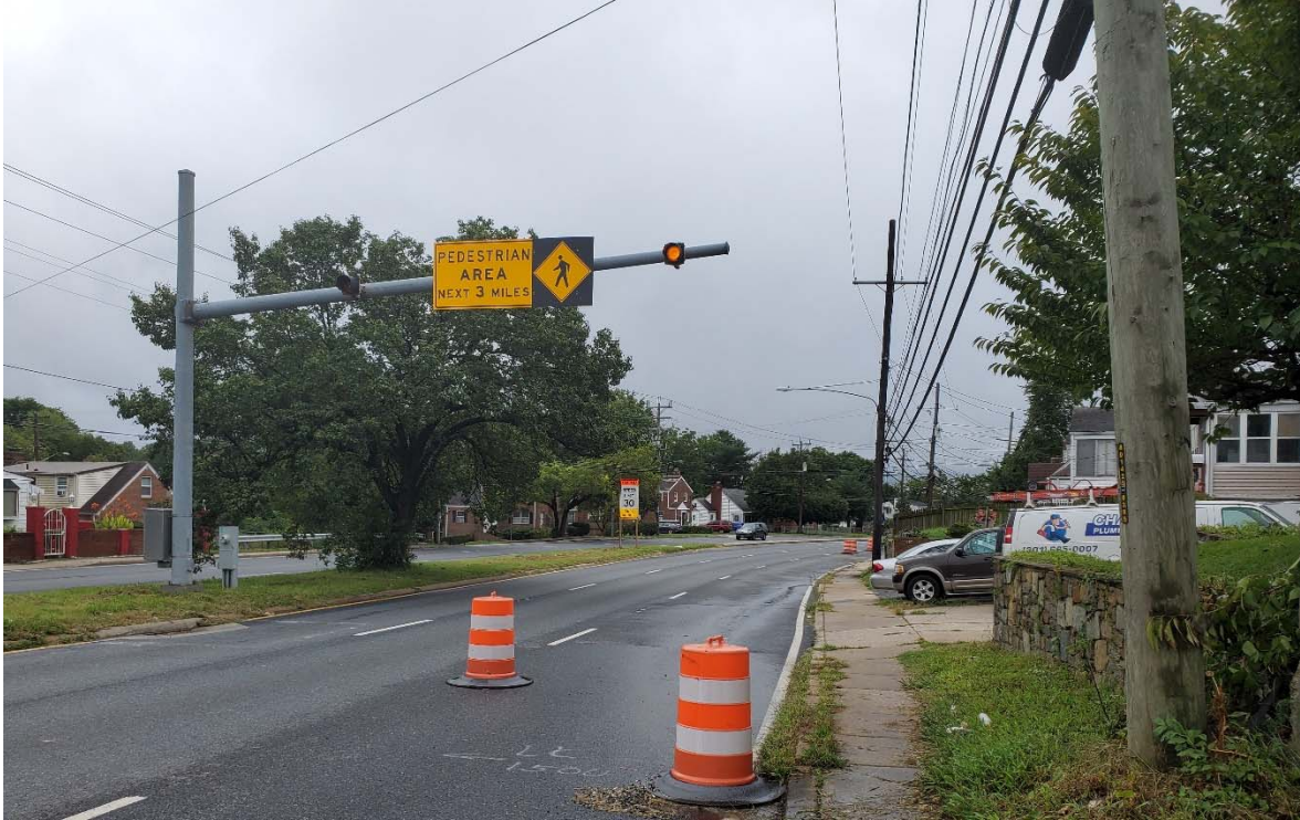
Picture 5: "Pedestrian Area Next 3 Miles" overhead sign with flashing beacons west of intersection over eastbound lanes. Looking in the direction of the intersection.
