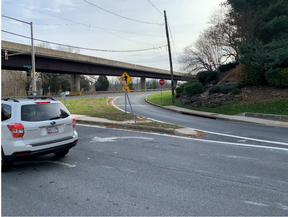
Picture 17: Stop-controlled slip lane at west leg of intersection.
