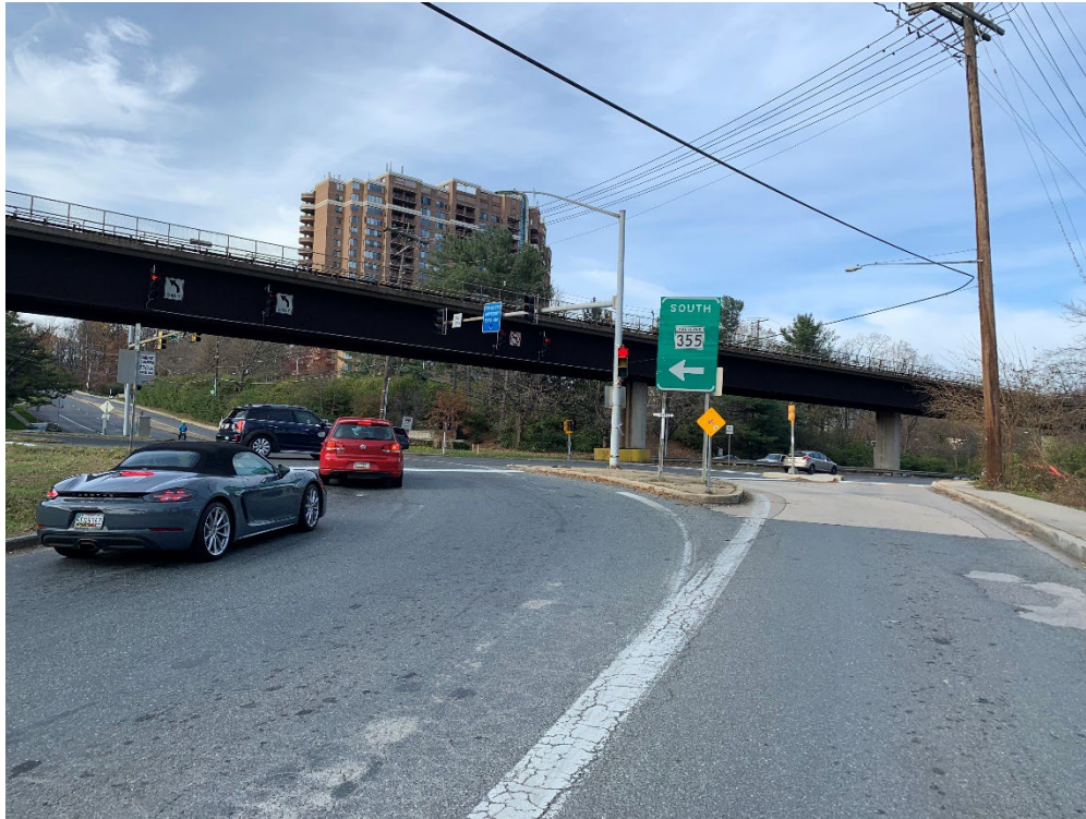
Picture 3: East leg of intersection facing MD 355.
