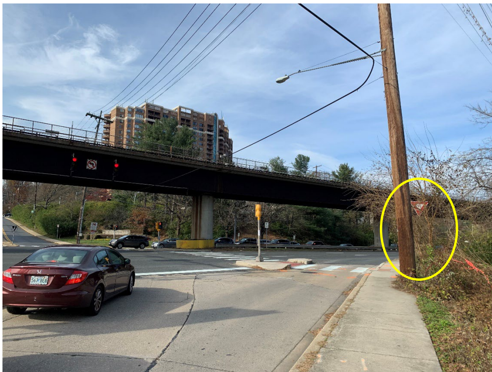
Picture 4: Slip lane to NB MD 355. Yield sign is blocked by foliage and utility pole (see yellow highlight).
