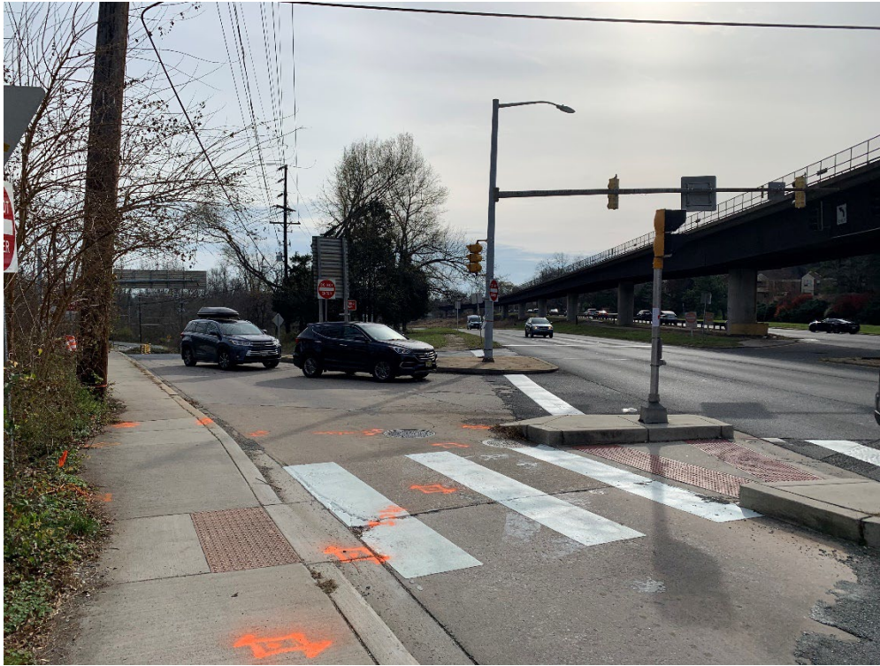
Picture 11: Crosswalk within slip lane at the NE corner of intersection.
