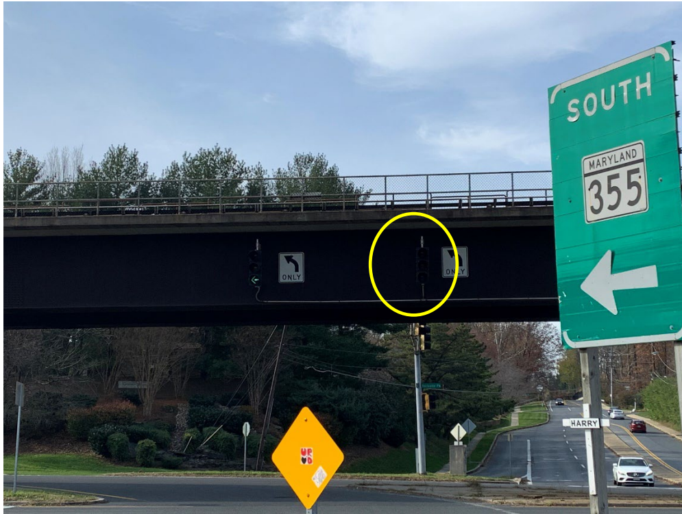
Picture 5: Signals facing east leg traffic. The green left turn signal is out (see yellow highlight).
