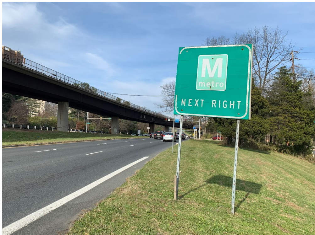
Picture 10: Faded “Metro, Next Right” sign with incomplete retroreflective border.
