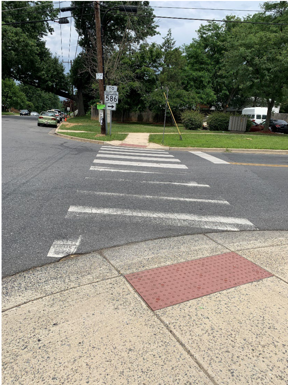
Faded Crosswalk – East Leg – Gridley Road
