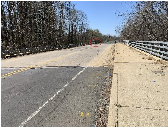
Westbound Norbeck Rd just at crash location
