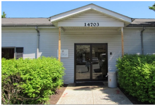
Figure 4. ARTC detoxification and intermediate care facility
