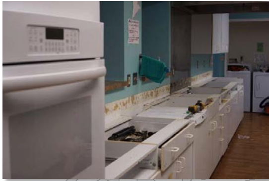
Figure 20. The reviewer panel was at WM during the renovations.
