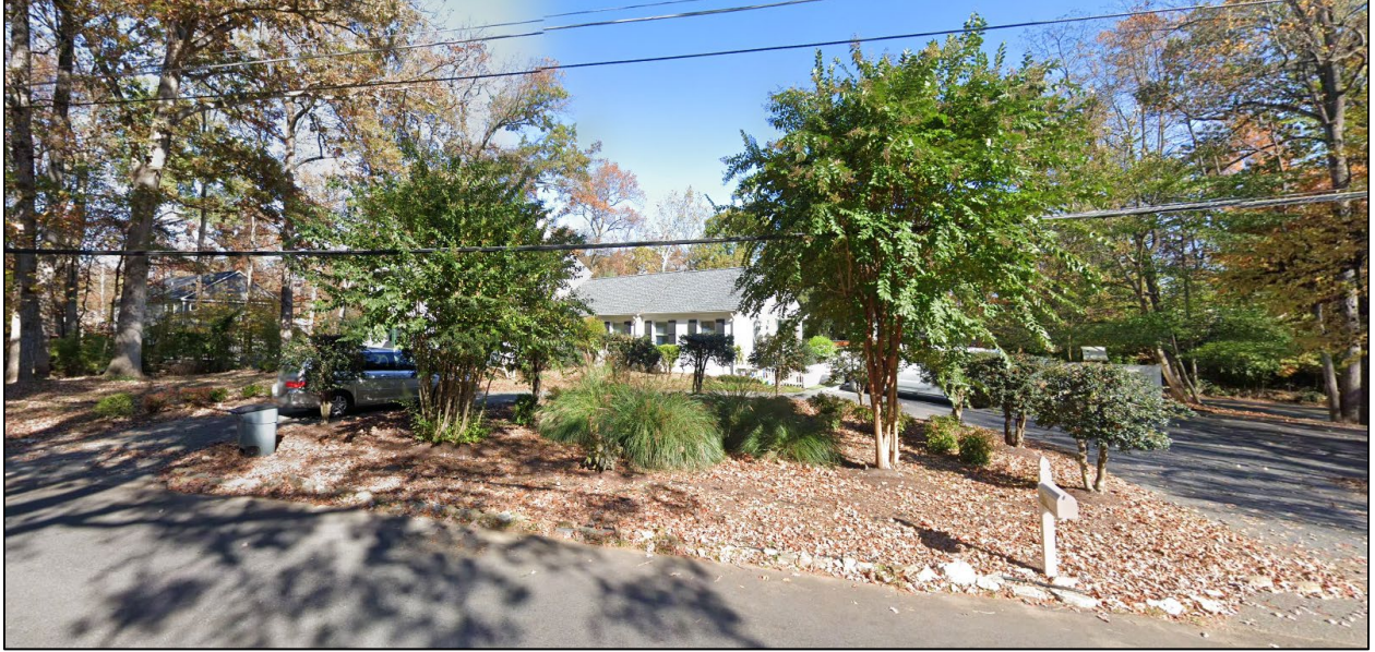
Figure 6: Front view of house, looking east from Greentree Road
