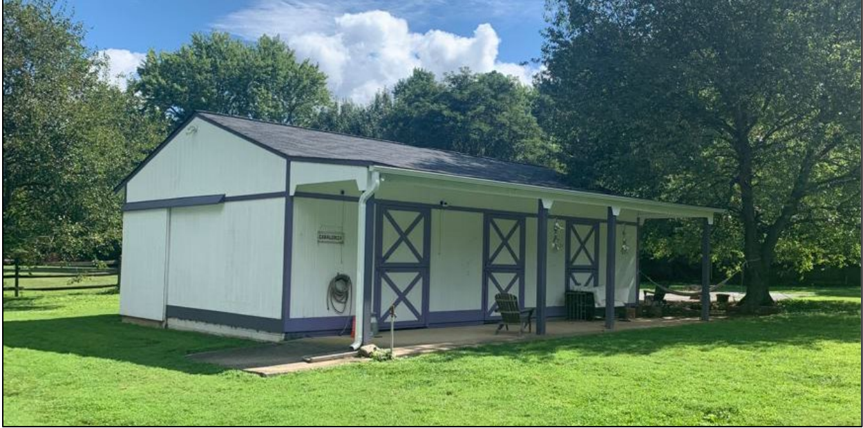
Figure 3. Existing barn on the Property (photo provided by Applicants)
