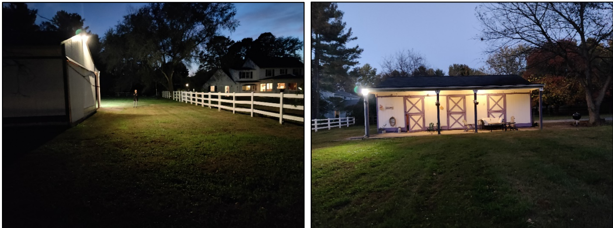
Figure 11. Existing lighting on barn: floodlights at tops of eaves on both ends (left) and under roof overhang in front (right). The picture on the left was taken from near the property line and shows that light from the floodlights does not spill onto the neighbor’s property. (Photos provided by Applicants)
