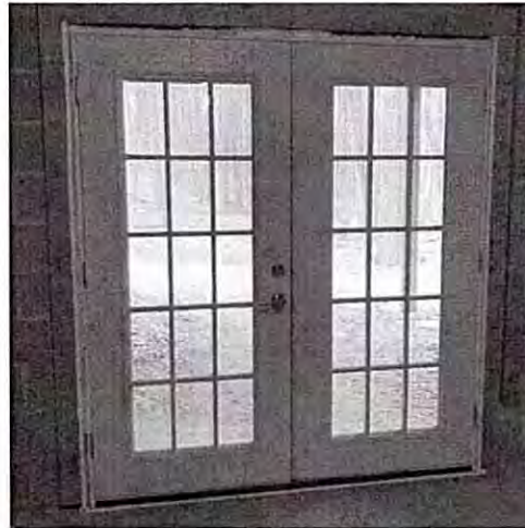
Figure 2: Exterior Basement Door
