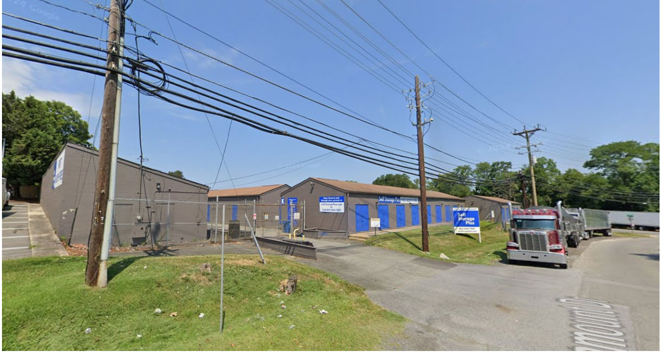
Figure 4: Street view from Paramount Drive, looking northwest.
