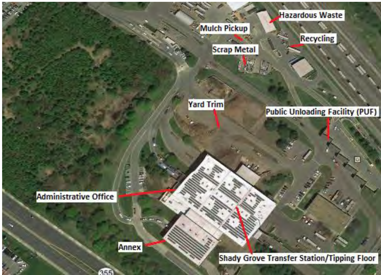
Figure ES 2 - Site Plan of Shady Grove Transfer Station and Processing Facility
