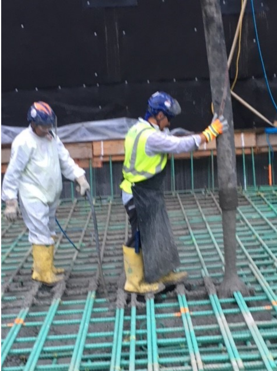
Advancing Voltex Waterproofing to Level P3
