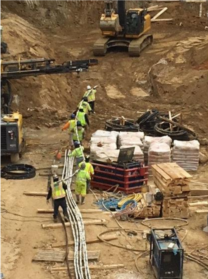
Workers Carrying Tie-Back Anchor to Installation Point
