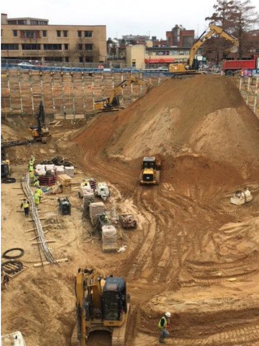
Excavators Working Together to Remove Excavated Material Uphill
