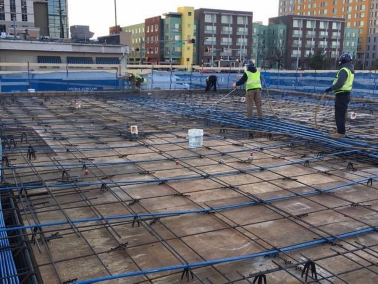
Second Floor Framing & Reinforcing - December 20, 2018
