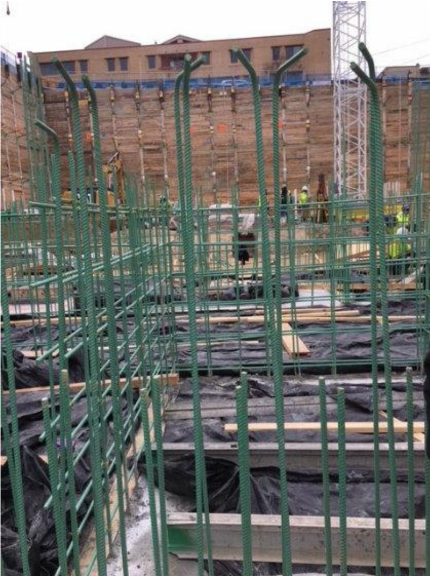
Reinforcing Below the Building Lobby
