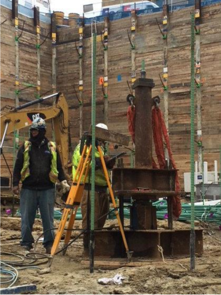
Hydraulic Testing a Tie-Down Anchor
