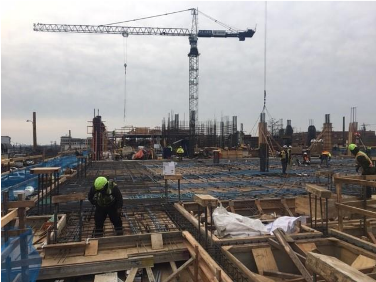
Photo showing typical floor construction - January 2019
