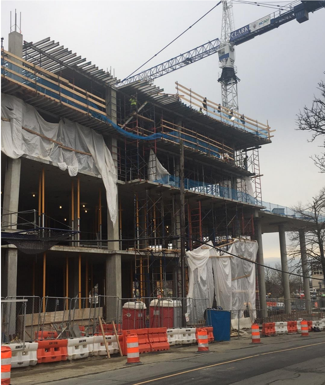
Fifth Floor under construction
