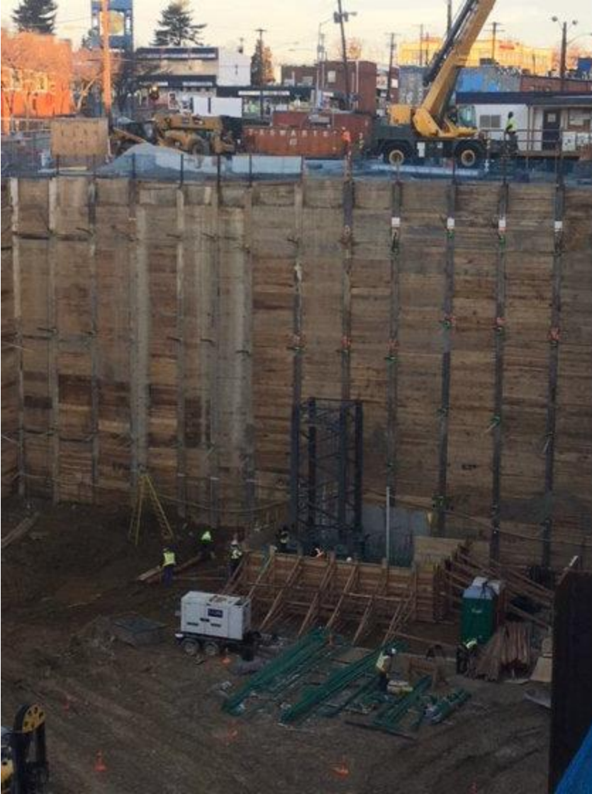
Foundation and Base for North Tower Crane
