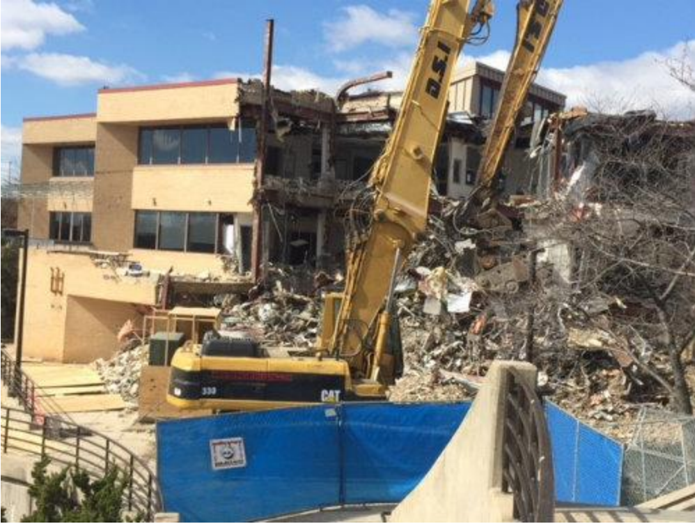
RSC Demolition Progress
