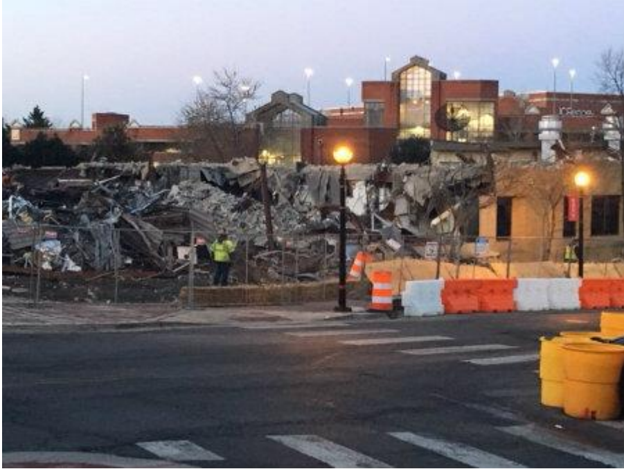
RSC Demolition Progress
