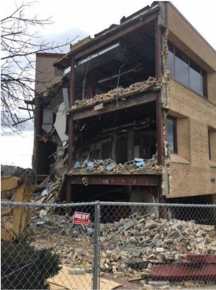
RSC Demolition Progress
