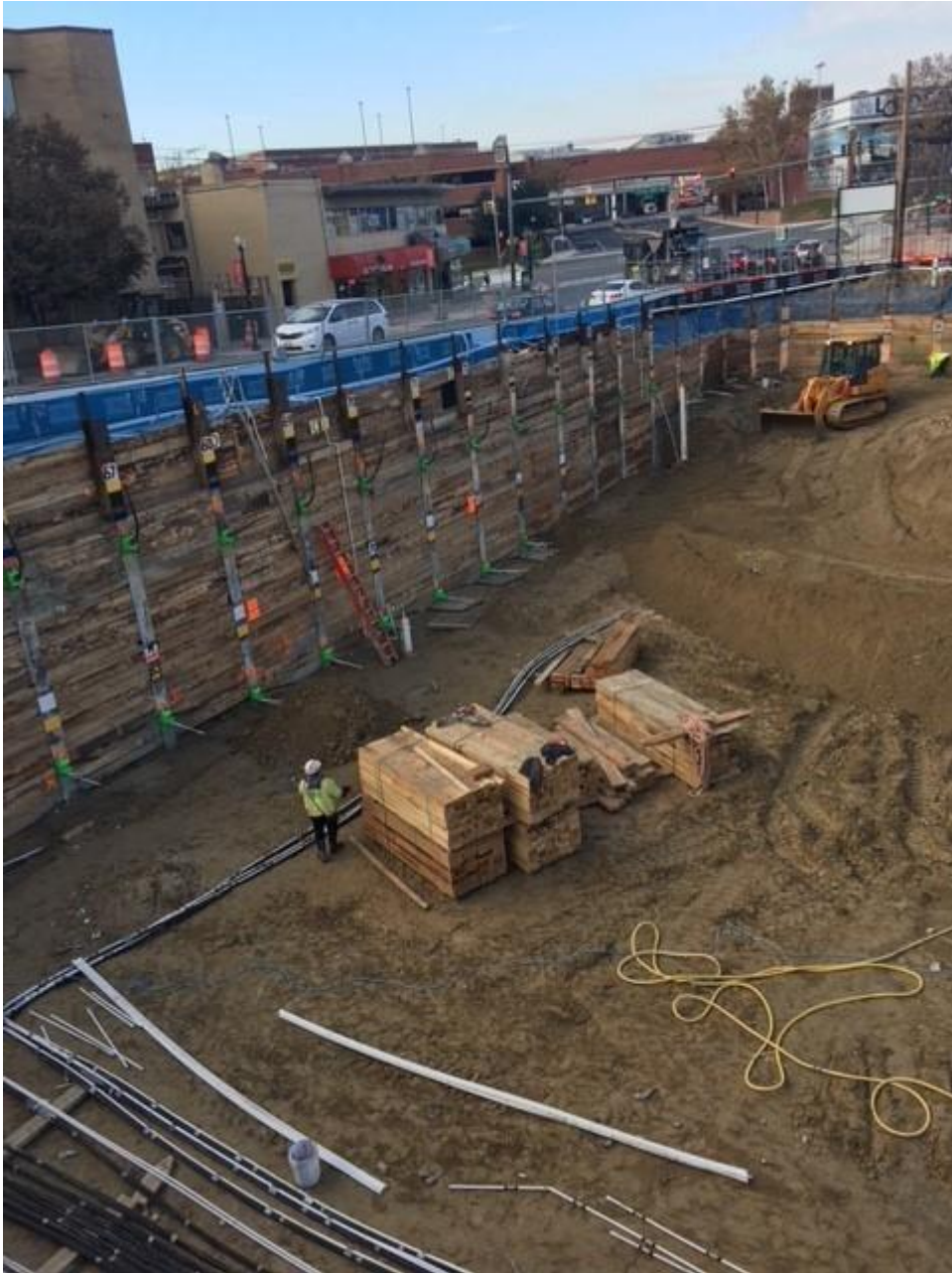
Excavation Advances along Triangle Lane
