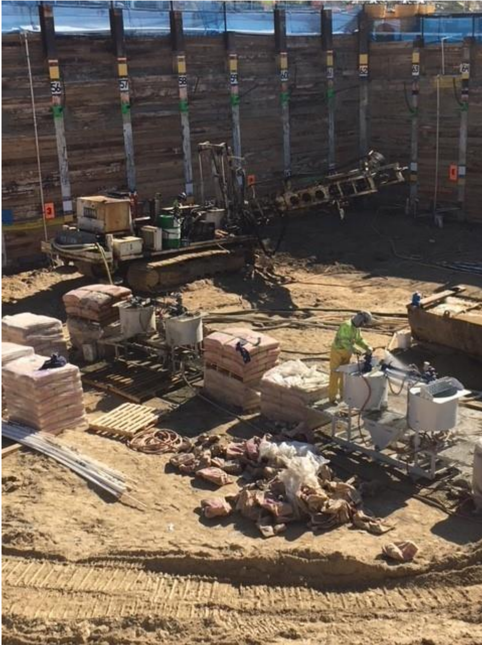
Tie Back Drill Rig (background)
