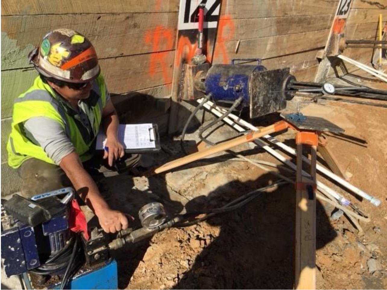
Hydraulic Jack-out Testing of Embedded Tie Back Anchor
