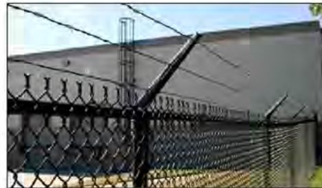
CHAIN LINK SECURITY FENCE
