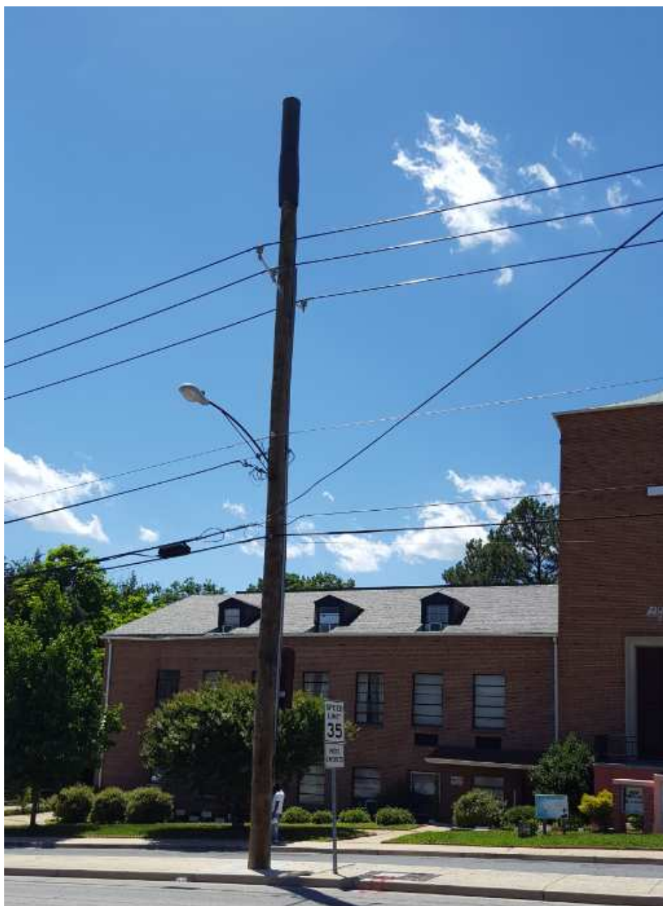
Figure 2: Photo of Small Cell Siting with 9.8 Cubic Feet of Equipment
