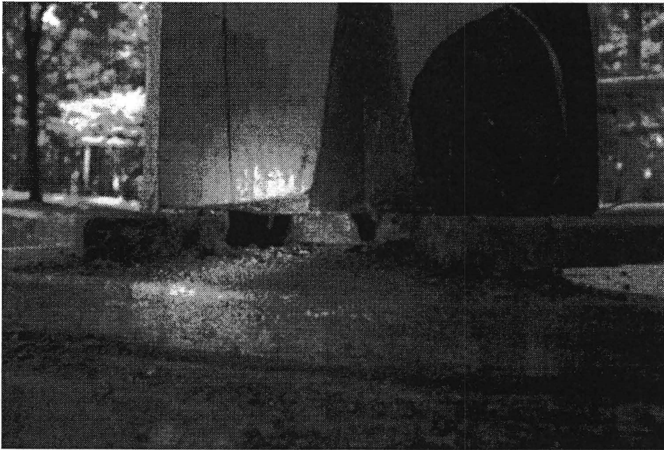
Steel I-beam support penetrating up into totem pole.
