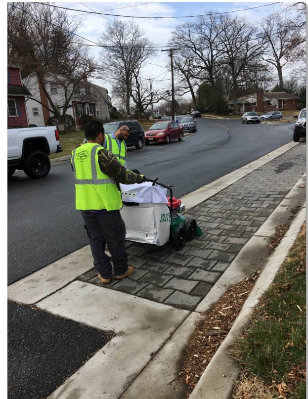
Pervious Pavement Cleaning
