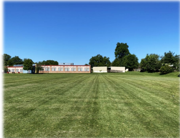
Harmony Hills Elementary School
