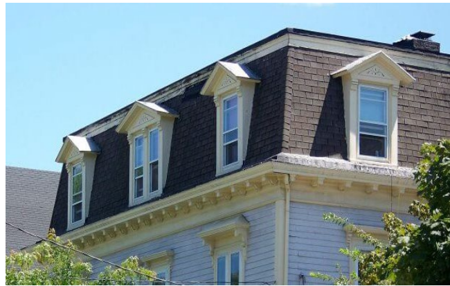
Figure 1a: Top Left Gable Roof Figure 1b: Top Right Hip Roof Figure 1c: Bottom Left Mansard Roof Figure 1d: Bottom Right Gambrel Roof
