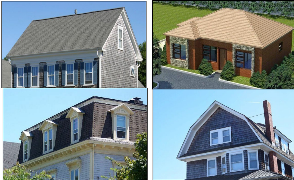
Figure 1a: Top Left - Gable Roof Figure 1b: Top Right - Hip Roof Figure 1c: Bottom Left - Mansard Roof Figure 1d: Bottom Right - Gambrel Roof
