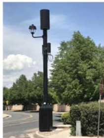
(b) A small cell attached at the top of a streetlight pole (Heilman, 2018).
