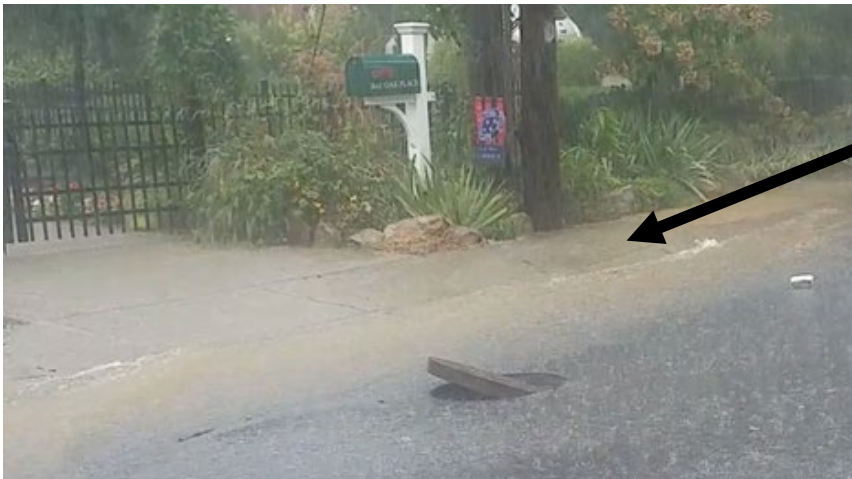
High-intensity events exceeding storm drain inlet capacity result in localized flooding impacts
