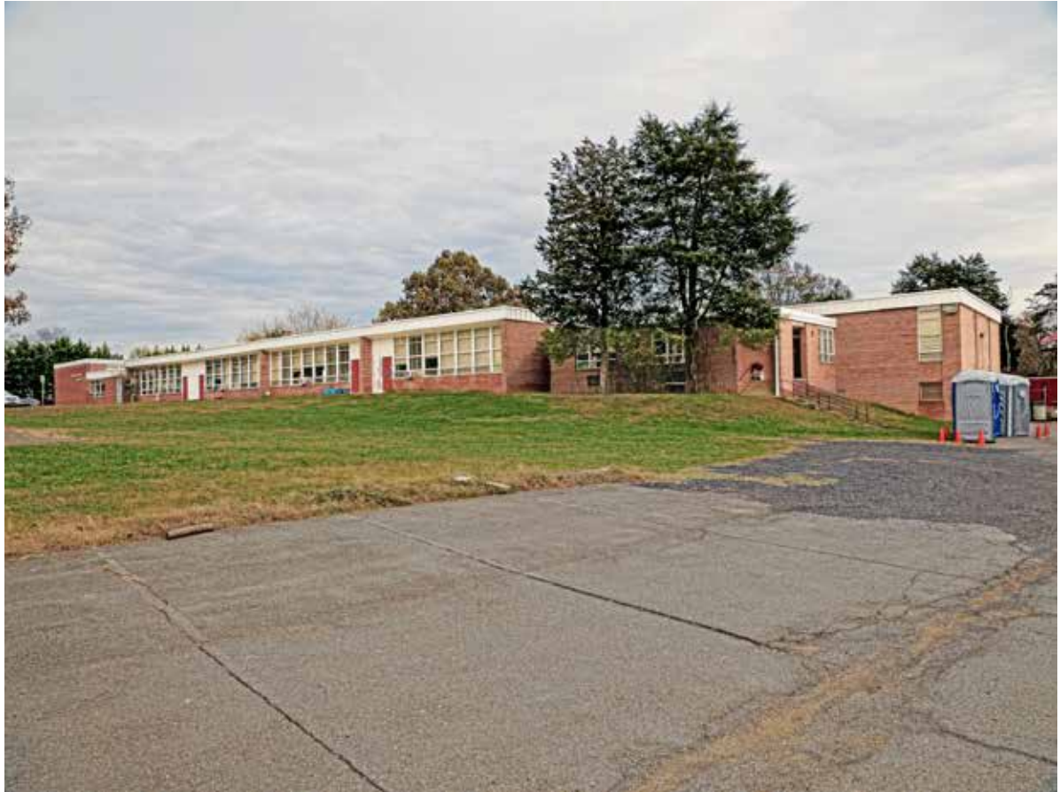
View of the Edward U. Taylor Elementary School showing the last addition. Source: Montgomery Planning
