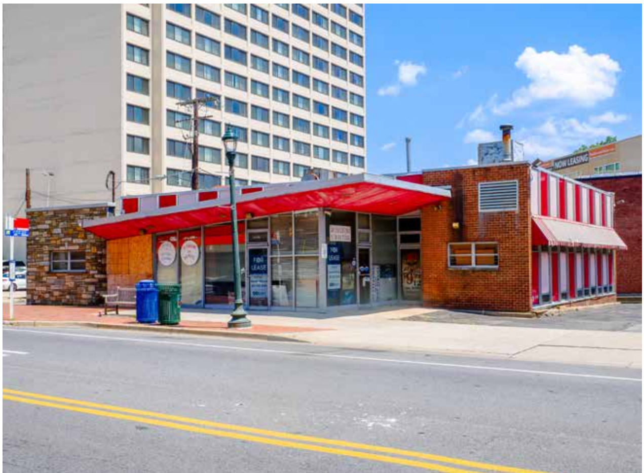
View of Weller's Dry Cleaning across Fenton Street, Summer 2022.
