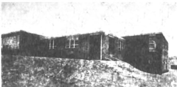
Photograph of the Taylor School's library and services wing, 1969.
