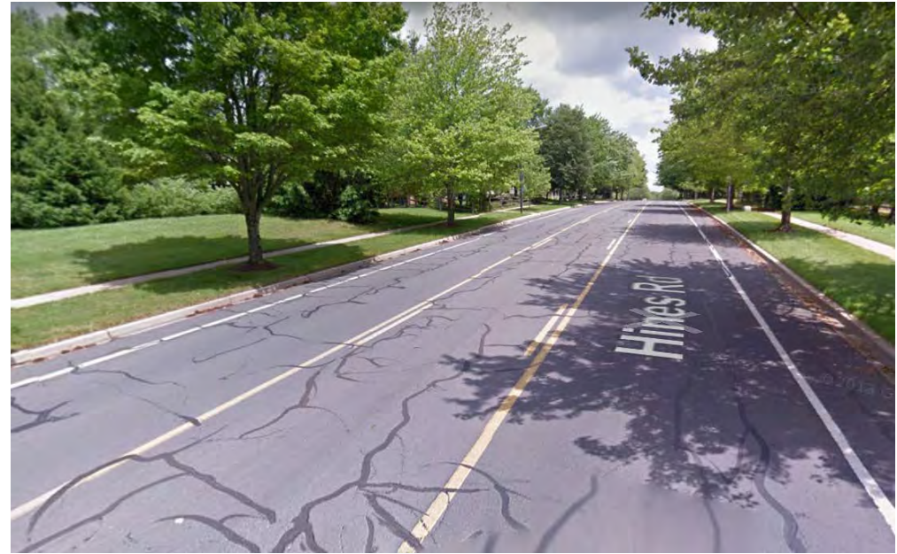
22. Views east and west along Hines Rd. Wide ROW and a striped turn lane offer opportunities to build either a buffered bike lane or separated bike lane.
