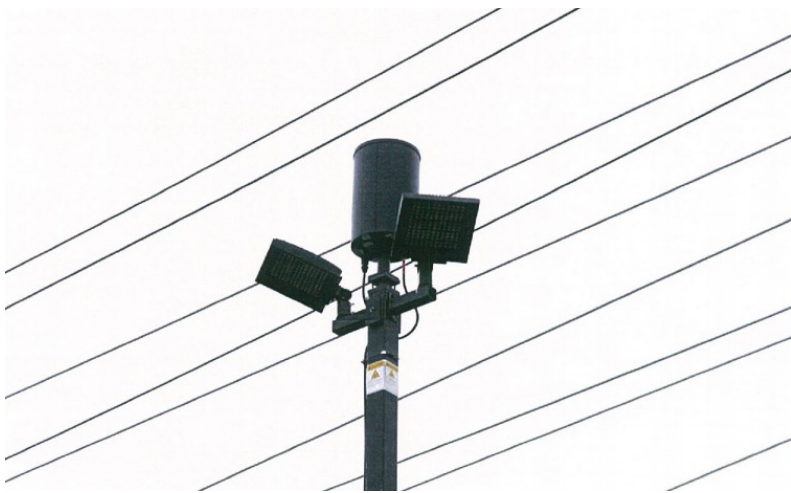
Existing small cell antenna in Rockville. Source: Bethesda Magazine.
