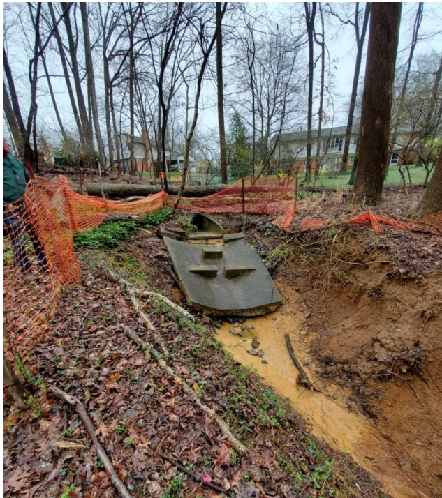
BEFORE – CONCRETE SPLASH PAD
