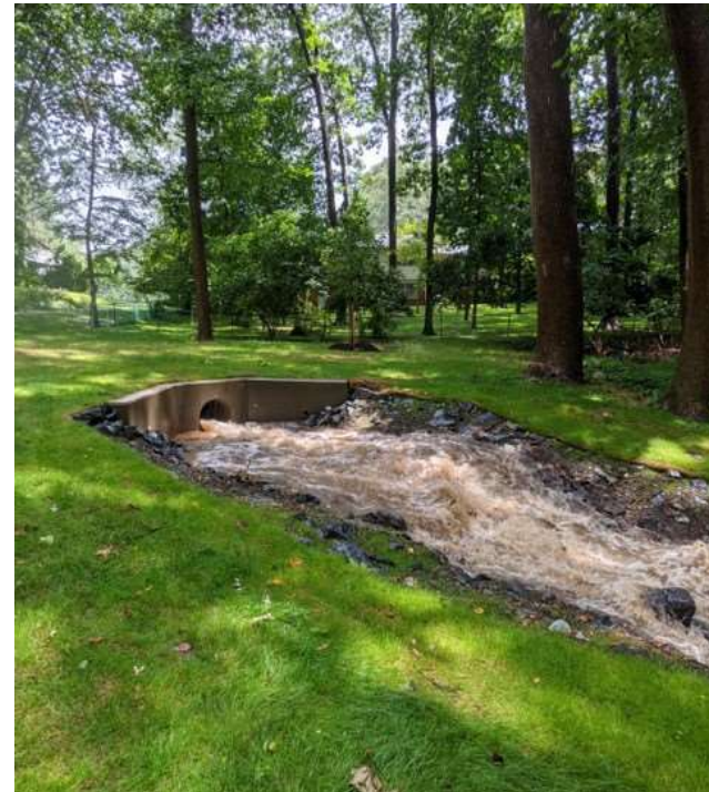
AFTER- ENDWALL AND PLUNGE POOL
