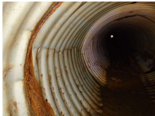
BEFORE 66" DIA. CMP (CORRUGATED METAL PIPE)
