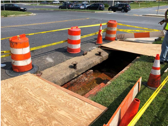
BEFORE – INLET – TOP REMOVED
