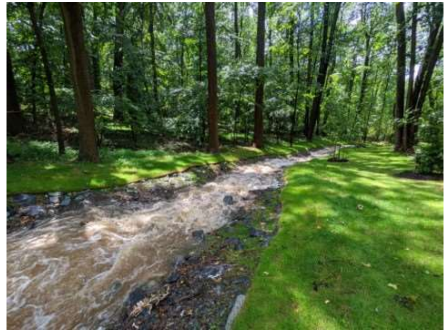
AFTER – STEP POOLS AND RIFFLE GRADE PROTECTION
