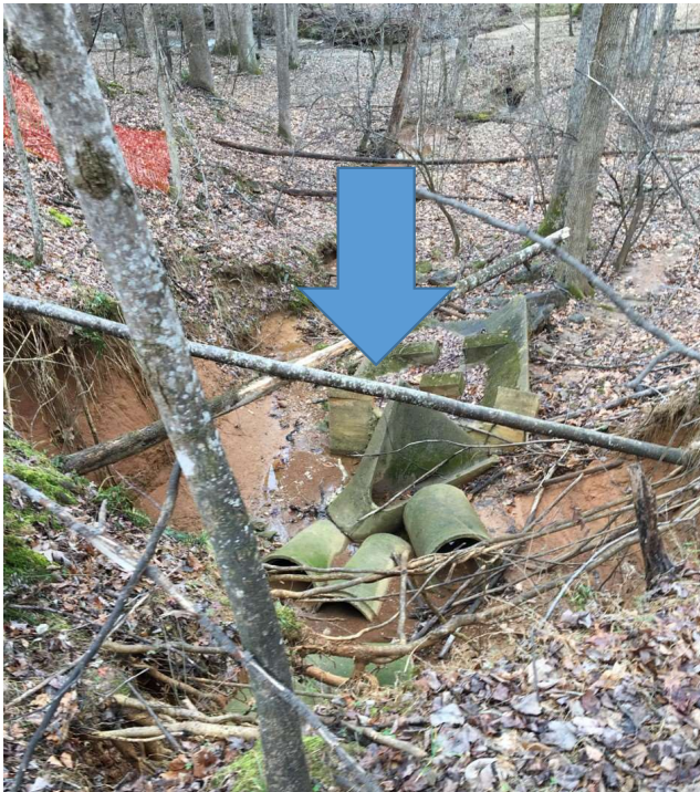
BEFORE – CONCRETE SPLASH PAD
