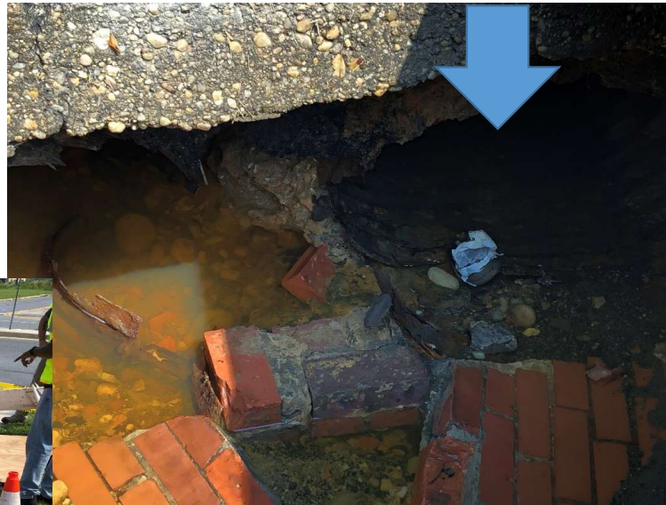
BEFORE – FAILED CMP STORM DRAIN AND BRICK INLET
