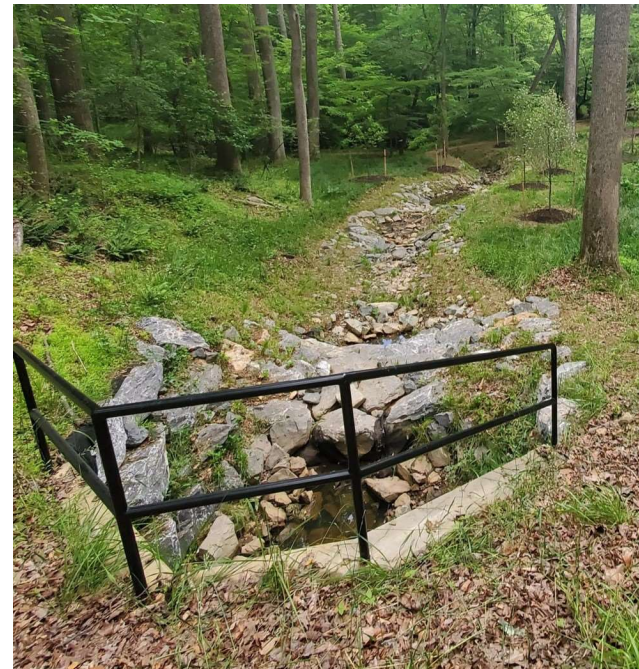
AFTER – ENDWALL WITH STEP POOLS
