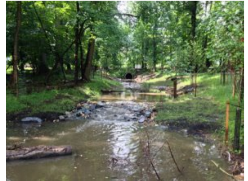
Breewood Stream Restoration After
