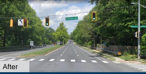
Signal changes at Shady Grove Rd & Briardale Rd with exclusive red turn phasing and backplates to address failure to yield crashes.
