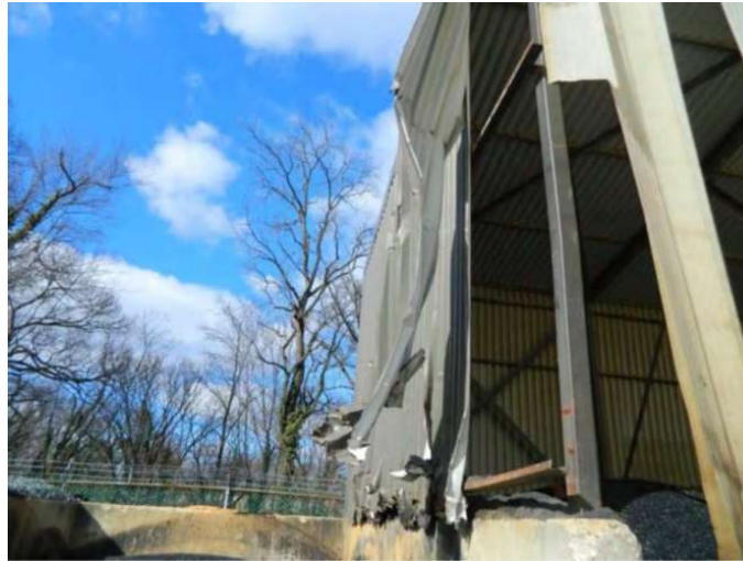
Gaithersburg Depot (deferred in FY 2023)
