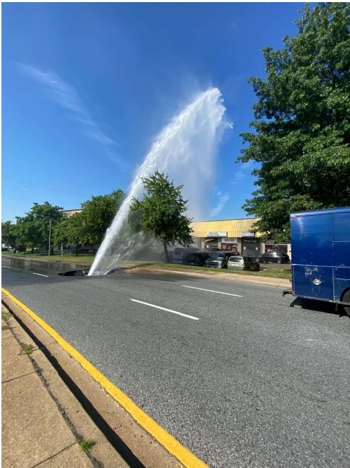
Capitol Heights Water Main Break July 2022
