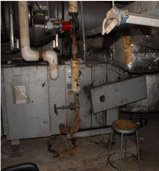
Anacostia Depot (deferred in FY 2023)
