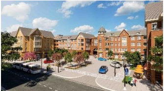
Avalon Somerville Station, Somerville, NJ - A 340 unit collection of mixed-use multifamily buildings integrated with the transit station nearing completion within the transit-oriented neighborhood in Somerville, NJ.
