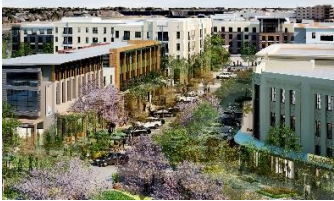
Midland Westridge Commons, Midland, TX - Creation of a regional destination for the Midland/Odessa market. The program includes retail, residential, office and hotel uses and is envisioned as a place for residents to live, work, play and gather with family and friends.
