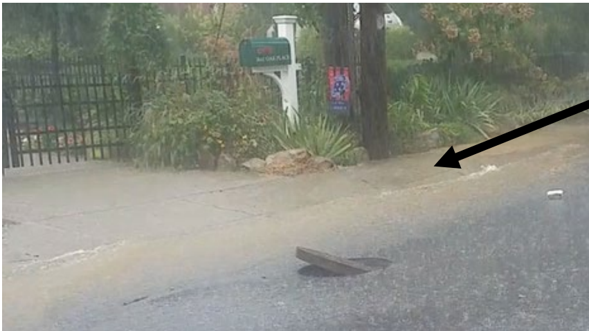
High-intensity events exceeding storm drain inlet capacity result in localized flooding impacts
